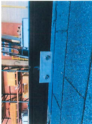
4. INSTALLATION IS COMPLETE WHEN THE BONDING HARDWARE PENETRATES THE OPPOSITE SIDE OF THE RAIL.
