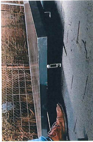
4. SEE MODULE ENGAGED BY ENDCLAMP.
