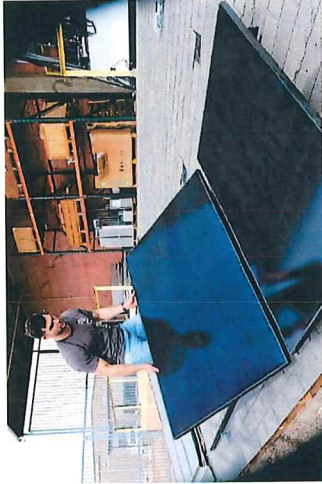
5. INSERT SECOND MODULE INTO PLACE.
