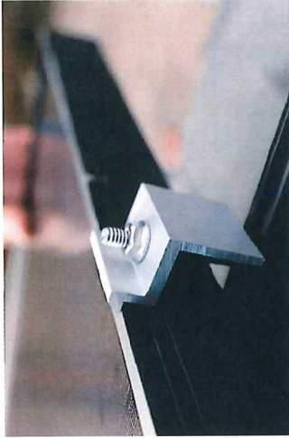
3. SEE MODULE ENGAGED BY ENDCLAMP.
