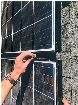
4. INSERT 1/4" T-BOLT INTO RAIL.
