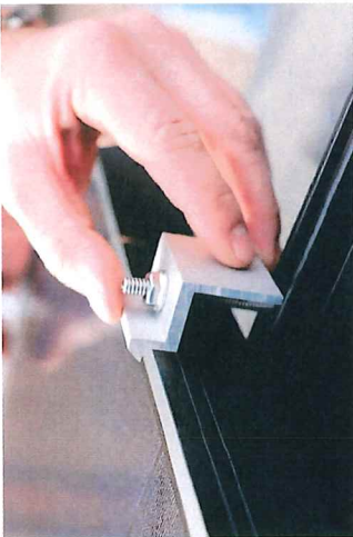
1. INSERT 1/4" T-BOLT INTO RAIL.
