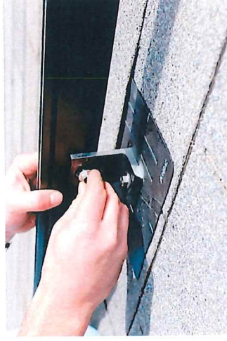
6. HAND TIGHTEN NUT UNTIL RAIL ALIGNMENT IS COMPLETE. VERIFY THAT POSITION INDICATOR ON BOLT IS VERTICAL (PER DRAWING 11.03.01.01.01).
