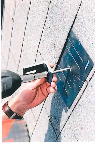
3. INSERT THE LAG BOLT THROUGH THE L-FOOT IN THE ORDER SHOWN IN THE IMAGE. VERIFY PROPER ORIENTATION BEFORE TIGHTENING LAG BOLTS.
