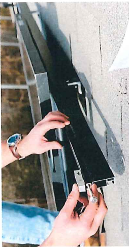
1. SLIDE END CLAMP ON TO RAIL BY ENGAGING THE TWO T-GUIDE BRACKETS WITH THE TOP SLOT OF THE RAILS. SLIDE END CLAMP ASSEMBLY ON TO RAIL UNTIL BOLT HEAD ENGAGES WITH END OF RAIL.
