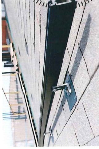
8. SEE RAIL ATTACHED TO L-FOOT.
