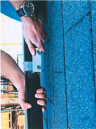
2. SLIDE T-FEATURE ON SPlice INTO THE T-SLOT ON EACH RAIL, CENTERING THE SPlice BETWEEN THE TWO RAILS.
