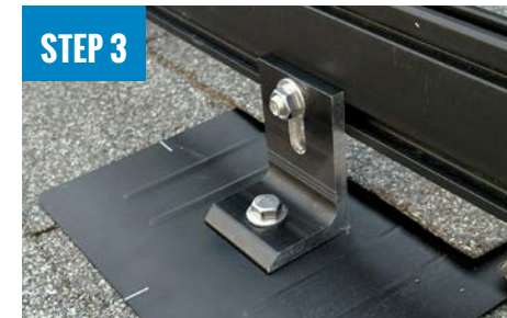
ATTACH L-FOOT TO RAIL
