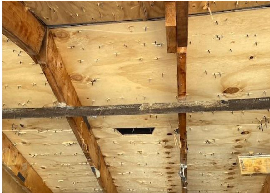
Photo No. 2 Underside Before Testing
