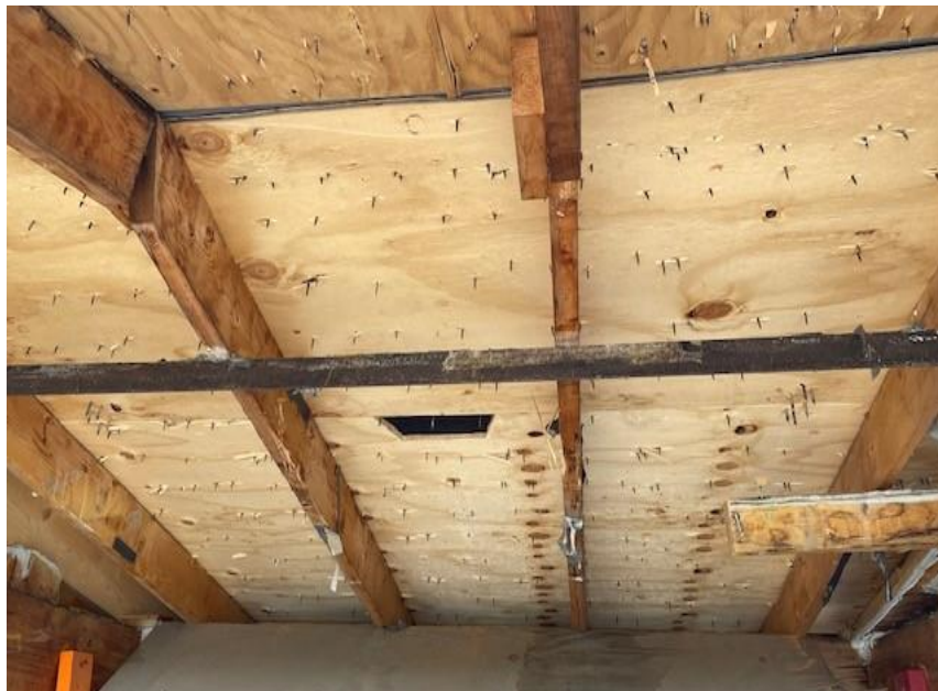
Photo No. 13 110 MPH Underside
