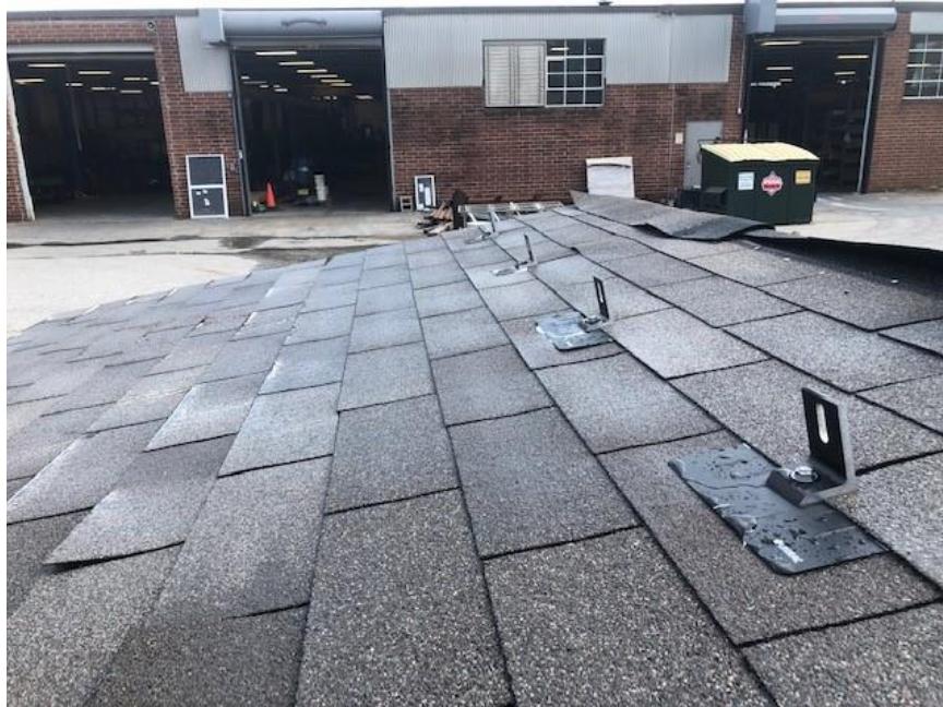
Photo No. 14 Post Test Top Side
