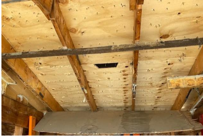
Photo No. 4 35 MPH Underside
