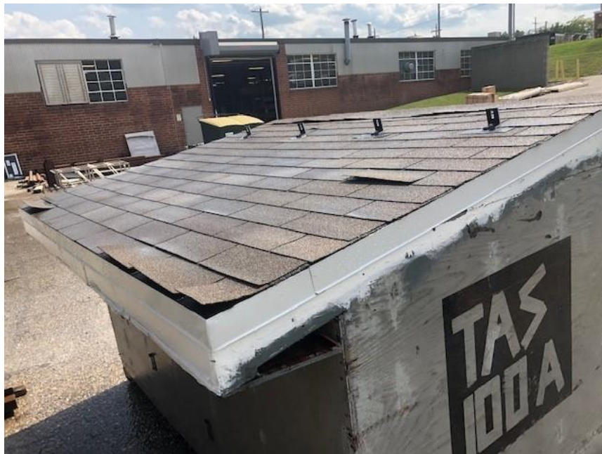
Photo No. 11 90 MPH Top Side After
