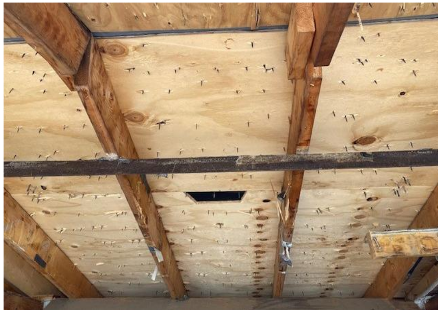
Photo No. 7 70 MPH Underside
