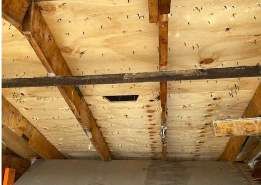
Photo No. 10 90 MPH Underside
