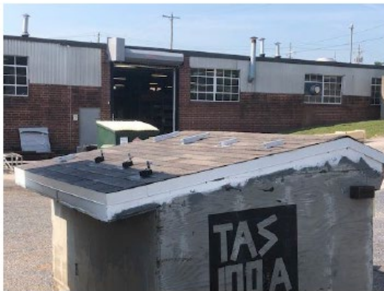
Photo No. 11 90 MPH Top Side After
