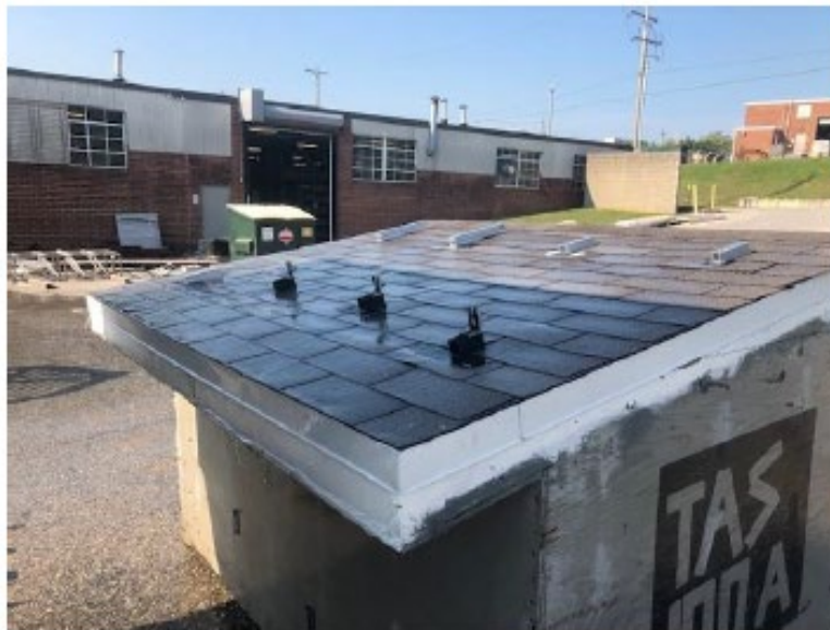
Photo No. 5 35 MPH Top Side After
