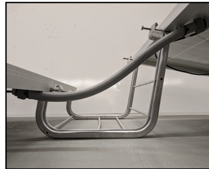
OPTION 3: USING FLEXIBLE NONMETALLIC CONDUITS
