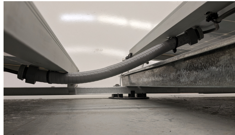
OPTION 2: USING FLEXIBLE NONMETALLIC CONDUITS
