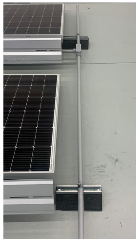
OPTION 2: USING RIGID NONMETALLIC CONDUITS
