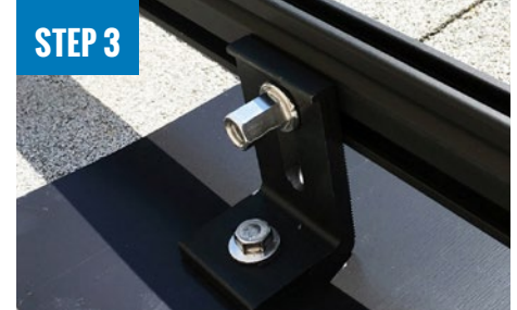
ATTACH L-FOOT TO RAIL
